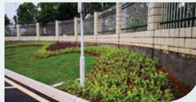
● Rain garden enables drainage of excessive rainwater, and at the same time beautify the area
